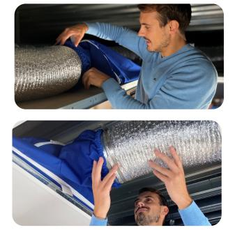
**Step 4** Connect the air supply and make sure the diffuser is properly seated.
