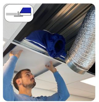
**Step 3** Place the diffuser into the open space, it is designed to fit precisely into the grid.
